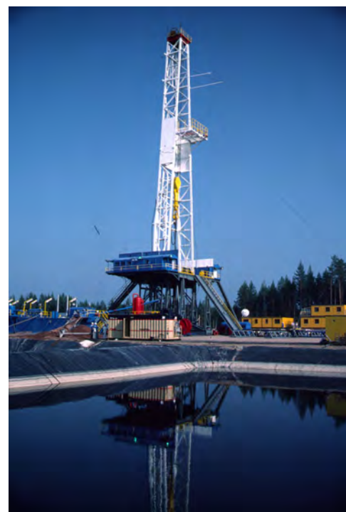
Figure 3. Heavy drilling rig suitable for deep borehole disposal
