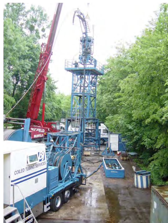
Figure 6. Coiled tubing unit
